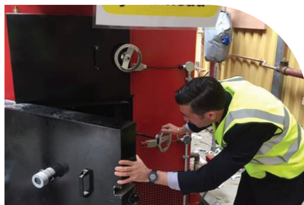
Fund Manager Bryn Jones inspects biomass boiler
